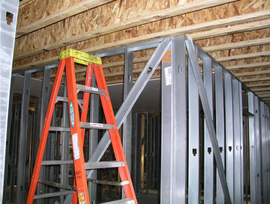
**Figure 4.1.1-3. Ceiling supports for experimental structure.**
